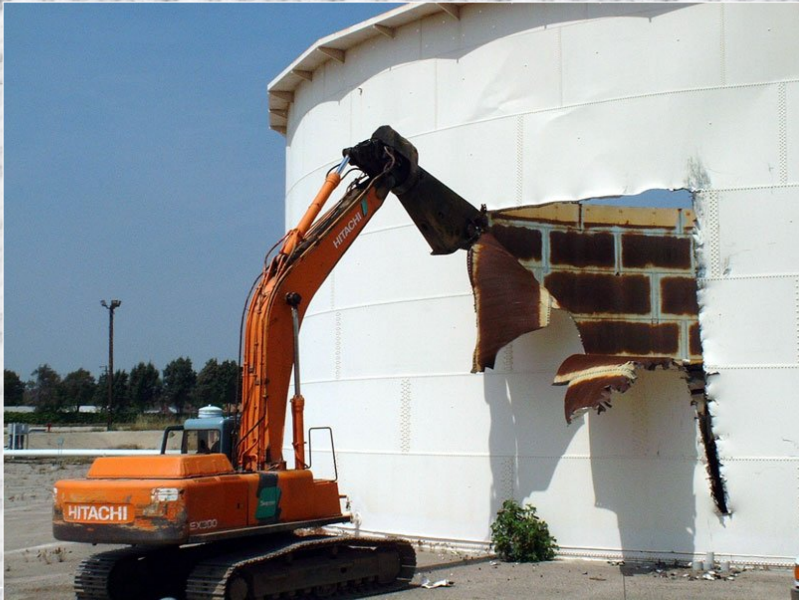
FIGURE 2 – SHEAR CUTTING FOR ACCESS
