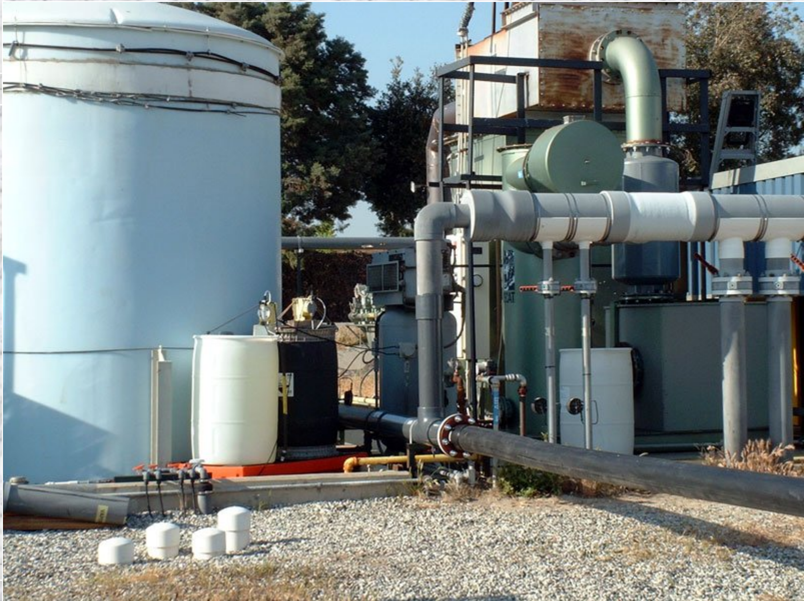
FIGURE 4 – FINAL CONNECTION TO SVE SYSTEM
