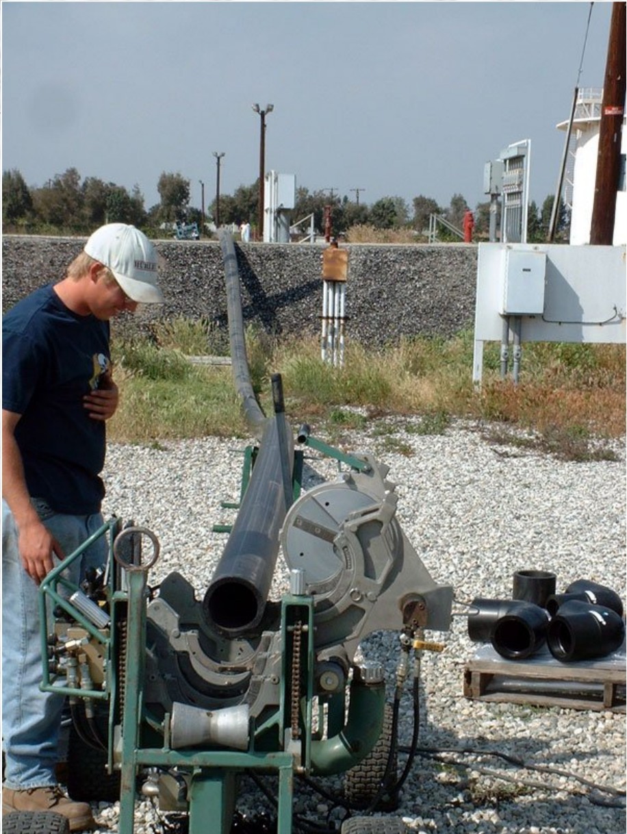
FIGURE 1 – HDPE PIPE INSTALLATION
